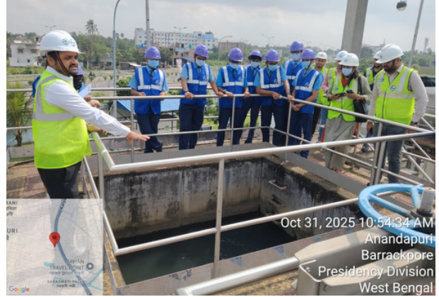
Assembly of God Church School visits the 18 MLD STP at Barrackpore
